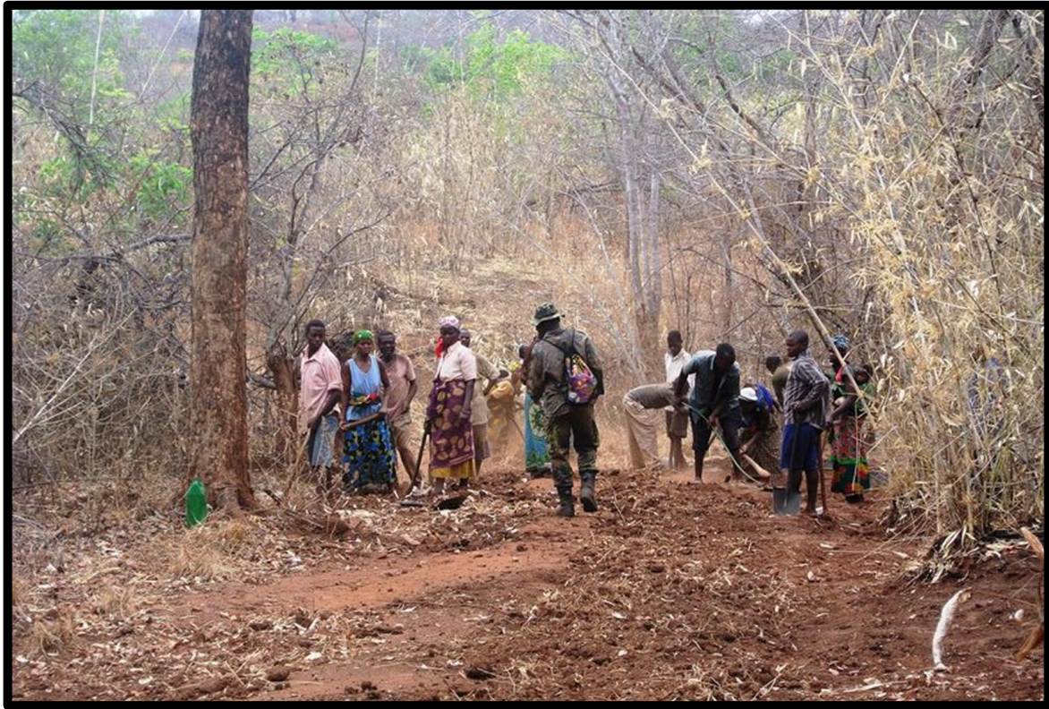
Road maintenance in Thuma
