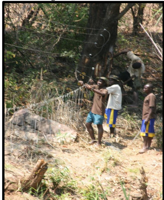
Adding chains to large ditch to stop elephants going under the fence
