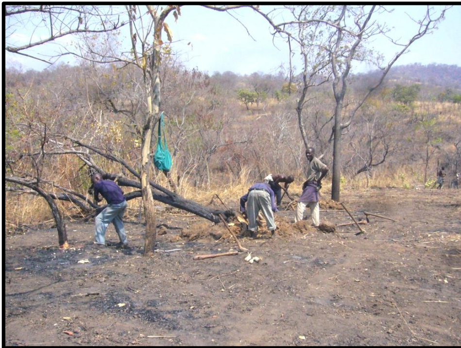
New fence line - Cutting trees
